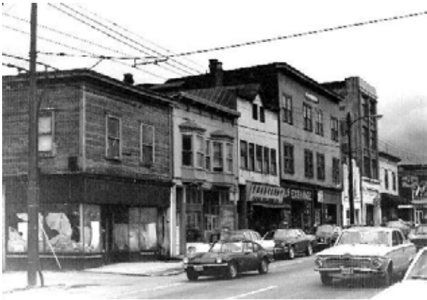
T. Matsumoto's building (second from the left), 235 Powell Street. Photo: Mike Hocevar (1975)
