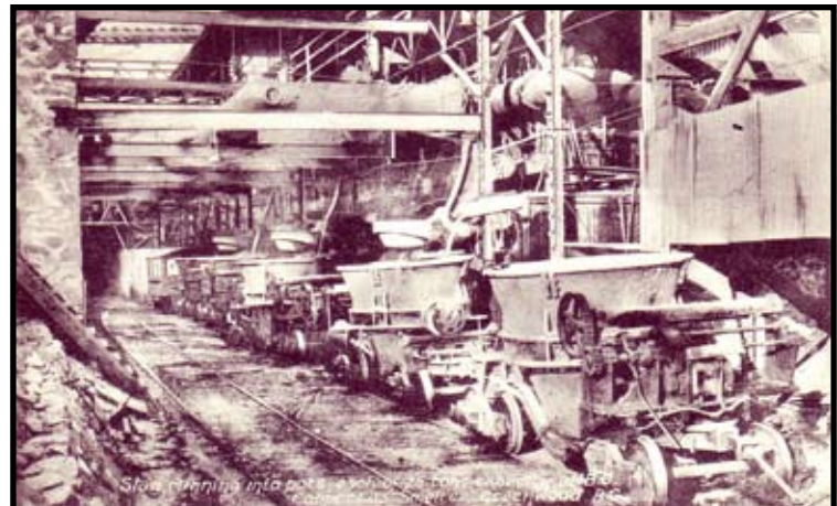
"Slag running into pots, each of 25 tons capacity at B.C. Copper Co.'s smelter, Greenwood, B.C." - Photo by McRae Bros.
