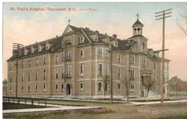
St. Paul's Hospital, Vancouver, B.C. Love Photo
